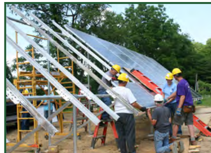
▲ 2011: Solar PV Workshop, Kutztown, PA
